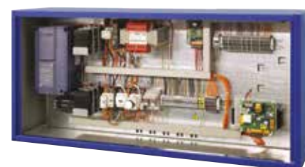
Power - Supply box
